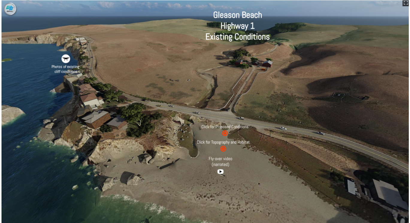
Aerial View of Existing Conditions
