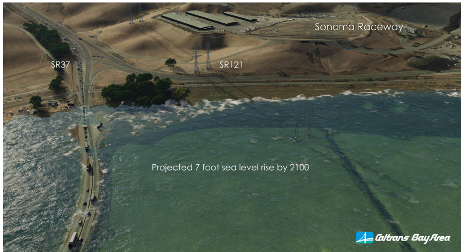
Projected Sea Level Rise over Existing Highway
